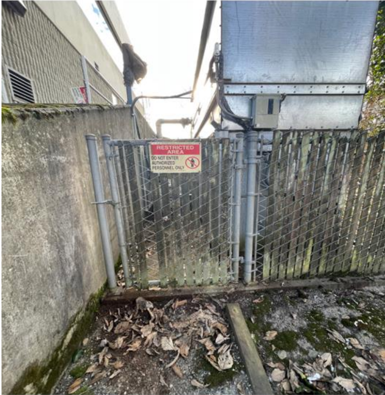
2. Cooling Tower view from North (looking south) ground level
